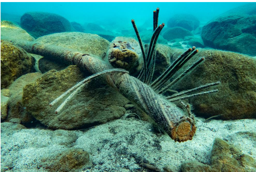
Submarine telecom cable
