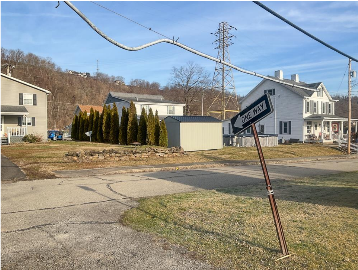
Lead cable sags between utility poles in Pennsylvania neighborhood Photo: Monique Rydel-Fortner
