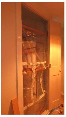
The airing cupboard had an old door that was warped as well as being painted, under the top layers, with lead paint. The door frame also had original lead paint.
