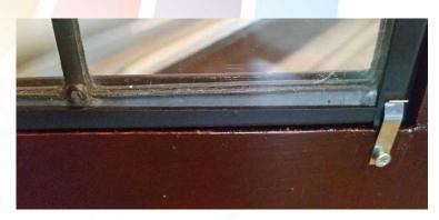
encapsulated panes were sealed with 40mm PVC tape and held in place with spring clips. Work on the windows was done away from the cabinets, with the windows placed in a cardboard box, while I was wearing PPE. The resultant encapsulation is almost invisible.
