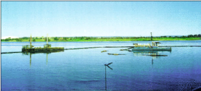
PHOTO: EGIS CONSULTING AUSTRALIA
