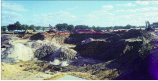
PHOTO: EGIS CONSULTING AUSTRALIA
