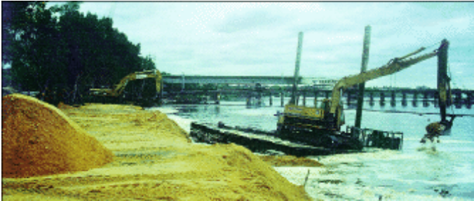
PHOTO: EGIS CONSULTING AUSTRALIA
